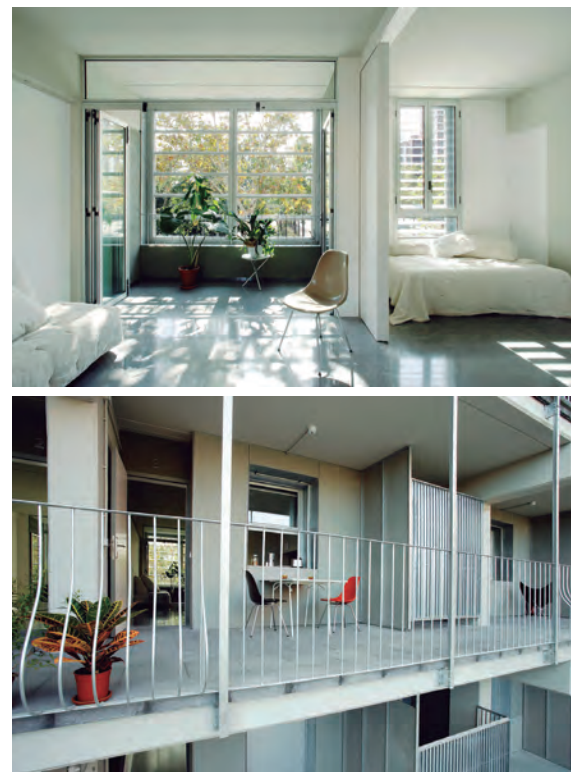
Figura 4.38 Viviendas para jóvenes en Sant Andreu. Arquitectos Emiliano López, Mónica Rivera, Guillermo Zuaznabar. Fuente: < https://lopez-rivera.com/project/competition-and-completion-of-housing-for-young-people-in-sant-andreu/ >
