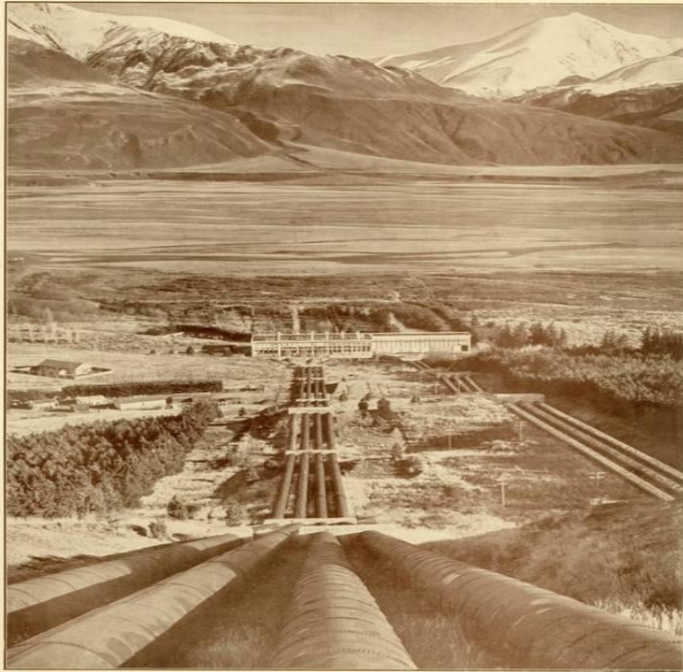
The Lake Coleridge Hydro-Electric Plant, showing the Rakai River, Tail Race, Power House and Pipe Lines. (65 miles west of Christchurch)
