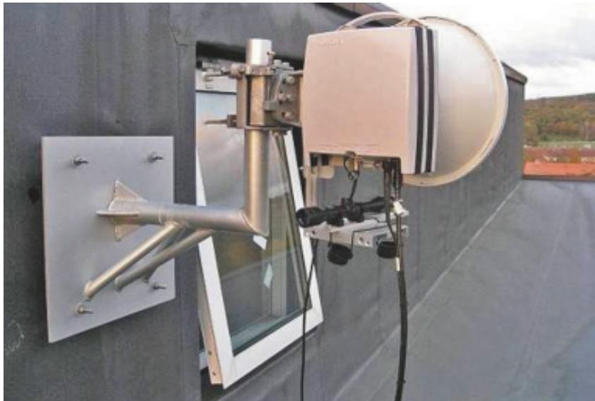
**Fig. 3** MMW dimensions, antenna diameter 39 cm (source: [5]).
