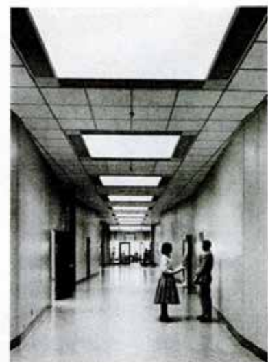
BRIGHT CORRIDOR, illuminated by overhead daylight, has zigzag walls to avoid monotony, echoes.
