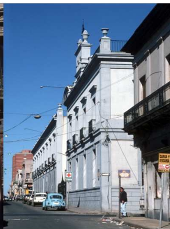
4. Hospital Maciel SMA-S073-004
