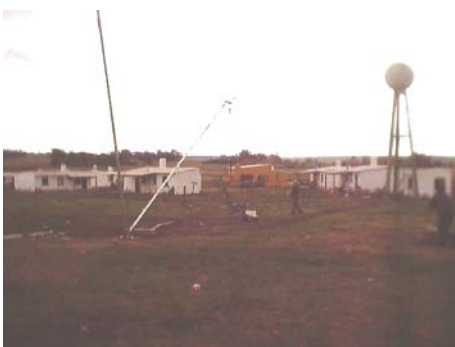
Fig. 8. Paso del Parque, Uruguay. Installation of the windmill
