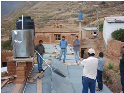
Fig. 4. Rodeo Colorado, Argentina. Community members working in the installation of solar water heaters.
