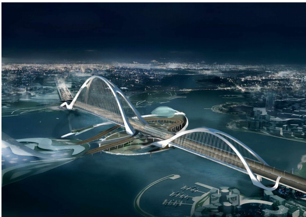
02. Sheikh Rashid bin Saeed Crossing- Foto: http://bit.ly_1AVnLvd.jpg
