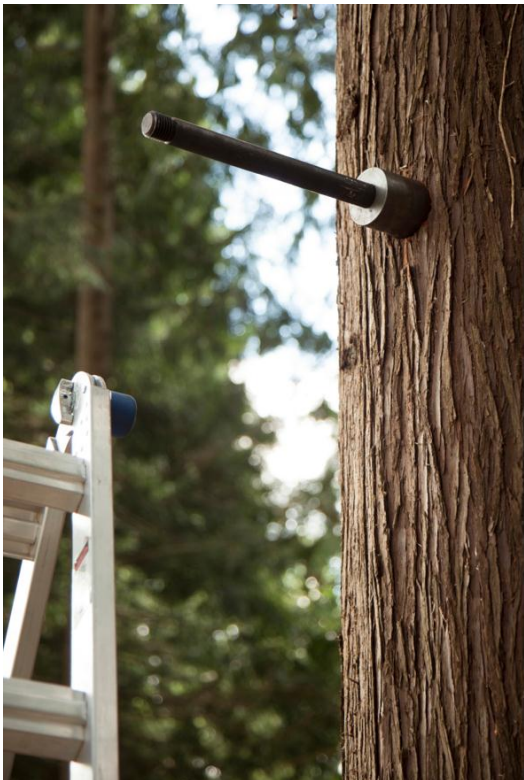
Anclaje deslizante. (Michael Garnier Out'n'About Treesort, < http://treehouses.com/joomla/LLC > (2012)
