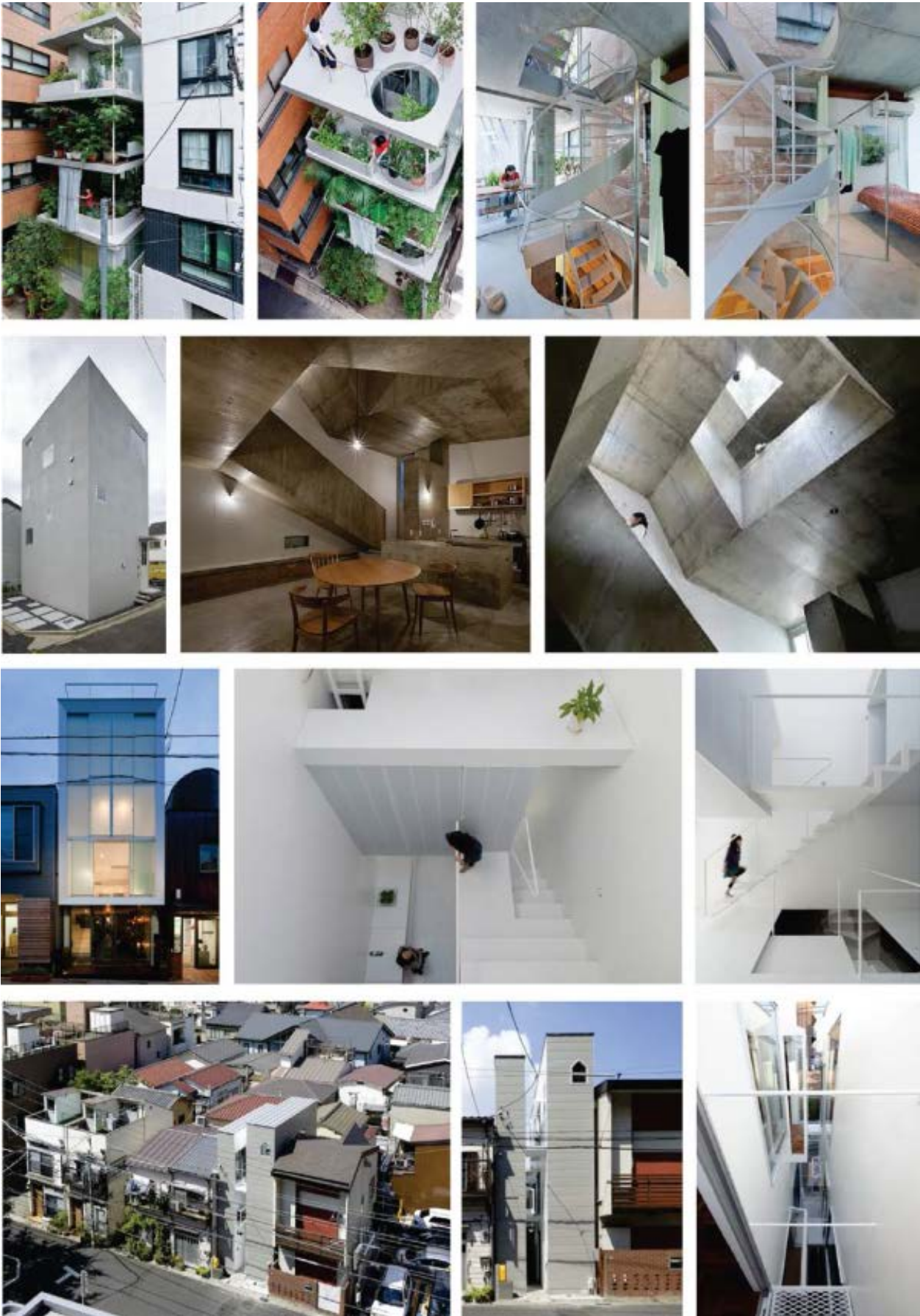
Ryue Nishizawa, Garden & House, Tokio - Suppose Design,- House in Nishiochiai, Nishiochiai - Makiko Tsukada, Kozuki House, Tokio - ON design, A life with a large opening, Tokio. Fotografías tomadas de sitios web, 2016.
